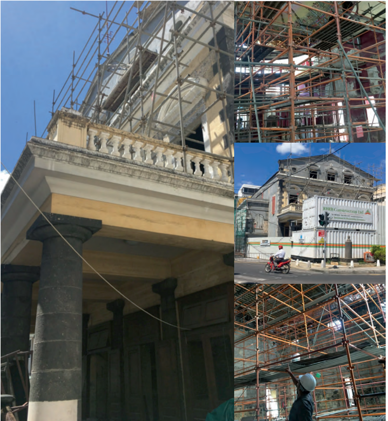
Renovation of Port Louis Theatre Phase I
