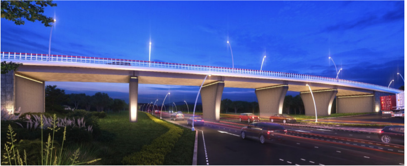
Flyover at Quay D Roundabout
