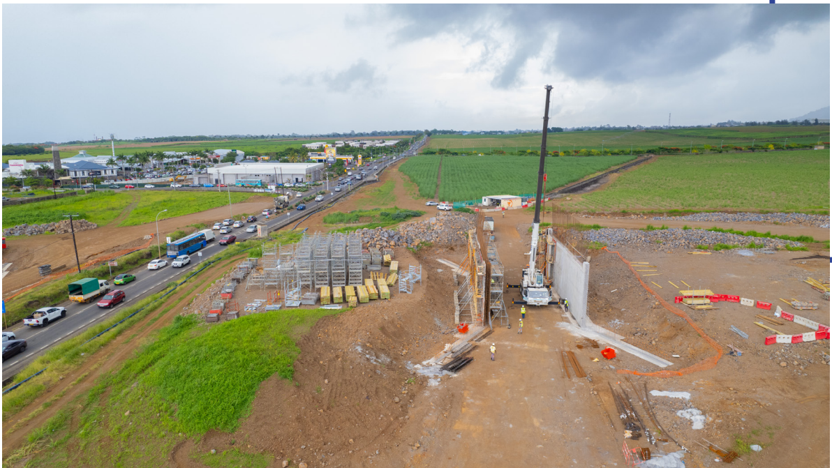
Construction of Flic-en-Flac Bypass from Xavier to Pierrefonds - RDA
