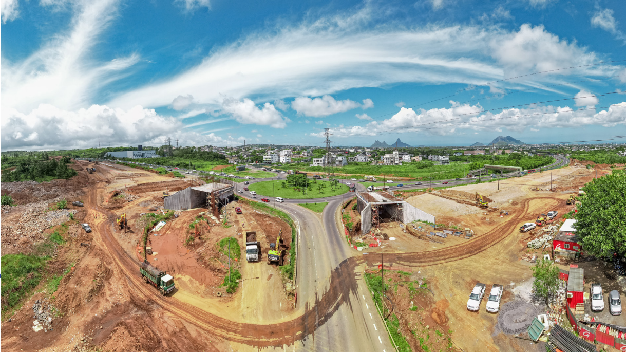
Design/Build/Turnkey for a Grade Separated Junction at Wooton - RDA
