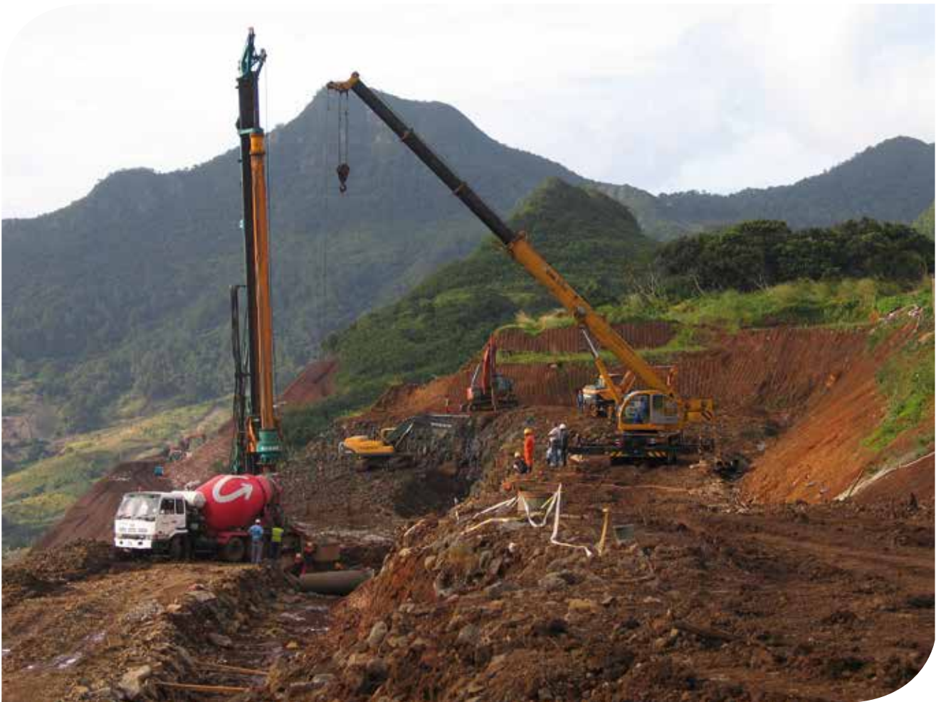
Treatment of Landslides at Ripailles – RDA
