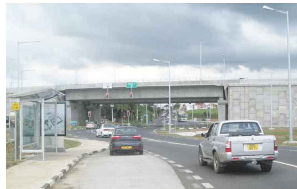
Figure 25: Fly-Over Bridge at Verdun
