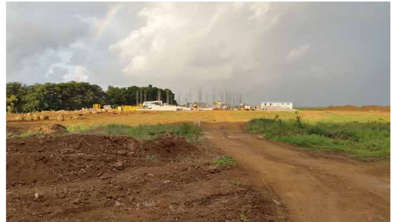
Figure 24: Construction Site – Pamplemousses University Campus
